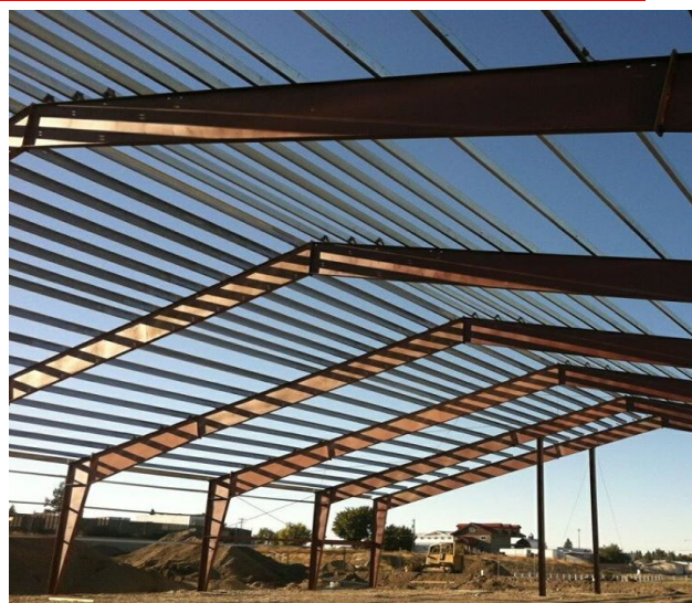
Structure Beams Taking Shape
